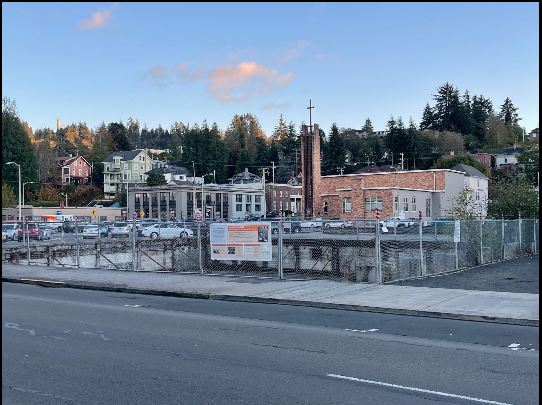
Heritage Square today Parking, Garden of Surging Waves, American Legion Hall
