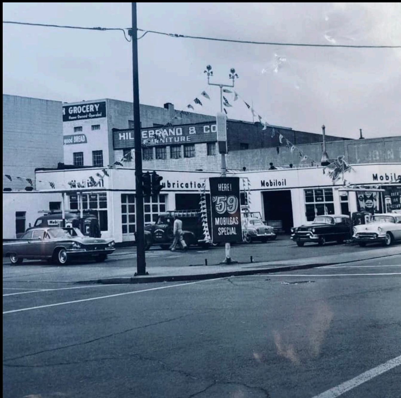
Mobil Gas/Service Station (c.1960) SE corner of 11 th and Duane Street
